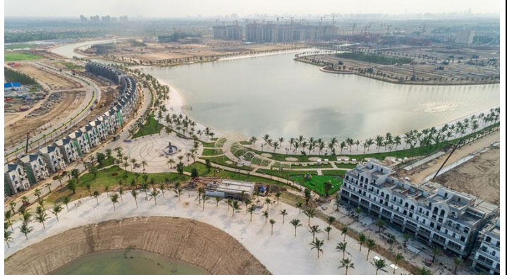
Figure 32: Ocean Park - The central reservoir and salt water lagoon were finished in 1H19
