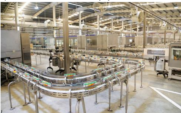
Figure 4: VNM’s mega factory is world’s most advanced dairy factory, which uses Tetra Pak’s technology. Around 90% of operation is handled automatically by robots
